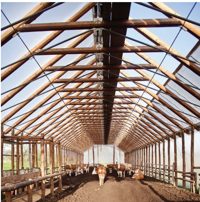
Figure 4. Barn for end-of-use disassembly and reuse of materials (Coop Tesori Bio farm, Cuneo, Piedmont, Italy).
